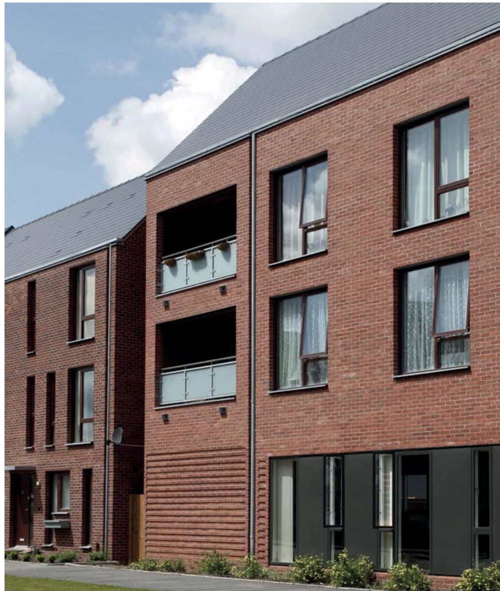
Red Facing Brick Used on 5 Keppel Street to clad the upper levels and provide a contextual connection to the existing buildings in the town centre
