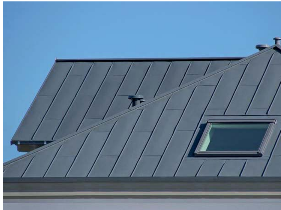
Folded Aluminium Roof Kalzip Falzinc or similar Used to clad the pitched roof on 5 Keppel Street as an alternative to slate and tile.
